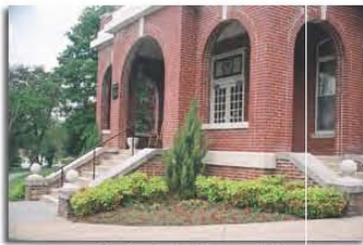
Main Building at VI
